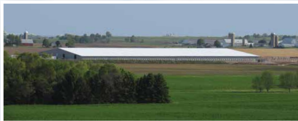
More than 70% of the roof on the new barn is up.
