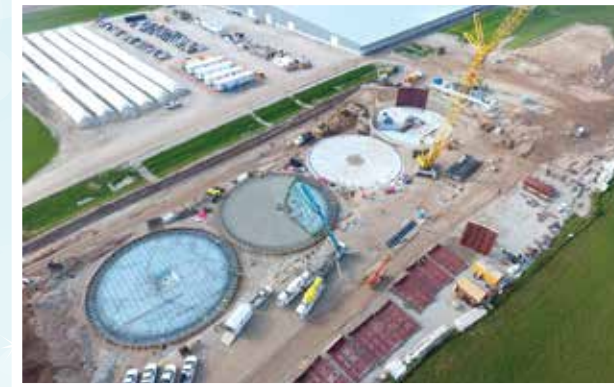
Aerial view of digester construction
